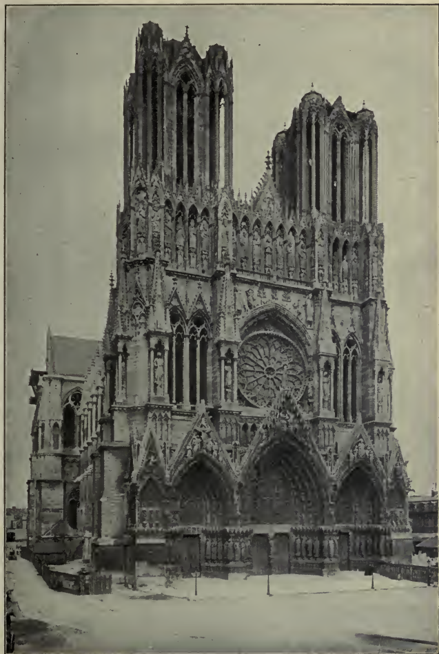
FAÇADE OF RHEIMS CATHEDRAL
